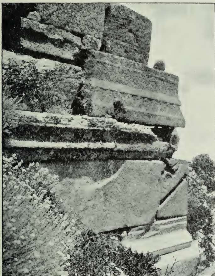
FIG. 282.—Kurshundju, monastery wall built of re-used stones.
